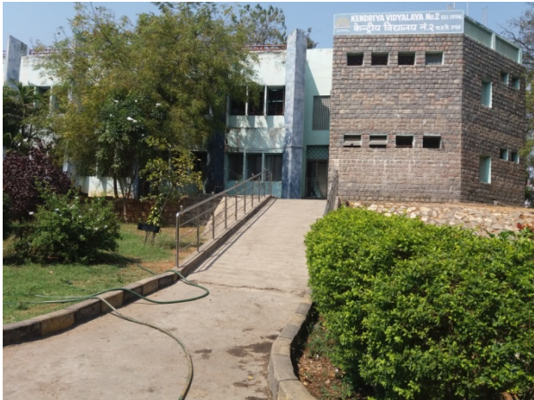
Fig 1 Stone Masonry Structure
